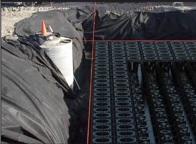
STRING LINES FACILITATE INSTALLATION OF BASE LAYER
