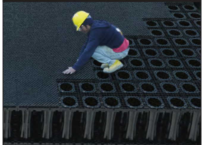
INSTALLING FLO-CELL® CAPPING LAYING OVER TANK MODULES
