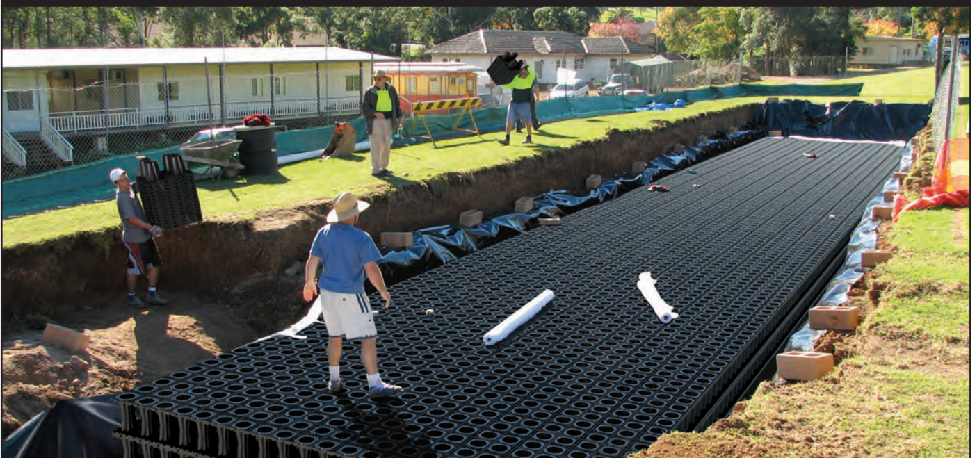
INSTALLING TANK MODULES
