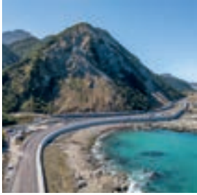
Rockfall and Landslide Embankments
