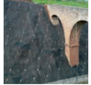
Flexible Structural Facing for Soil Nailing
