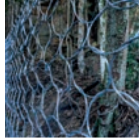
Dynamic Rockfall Barriers
