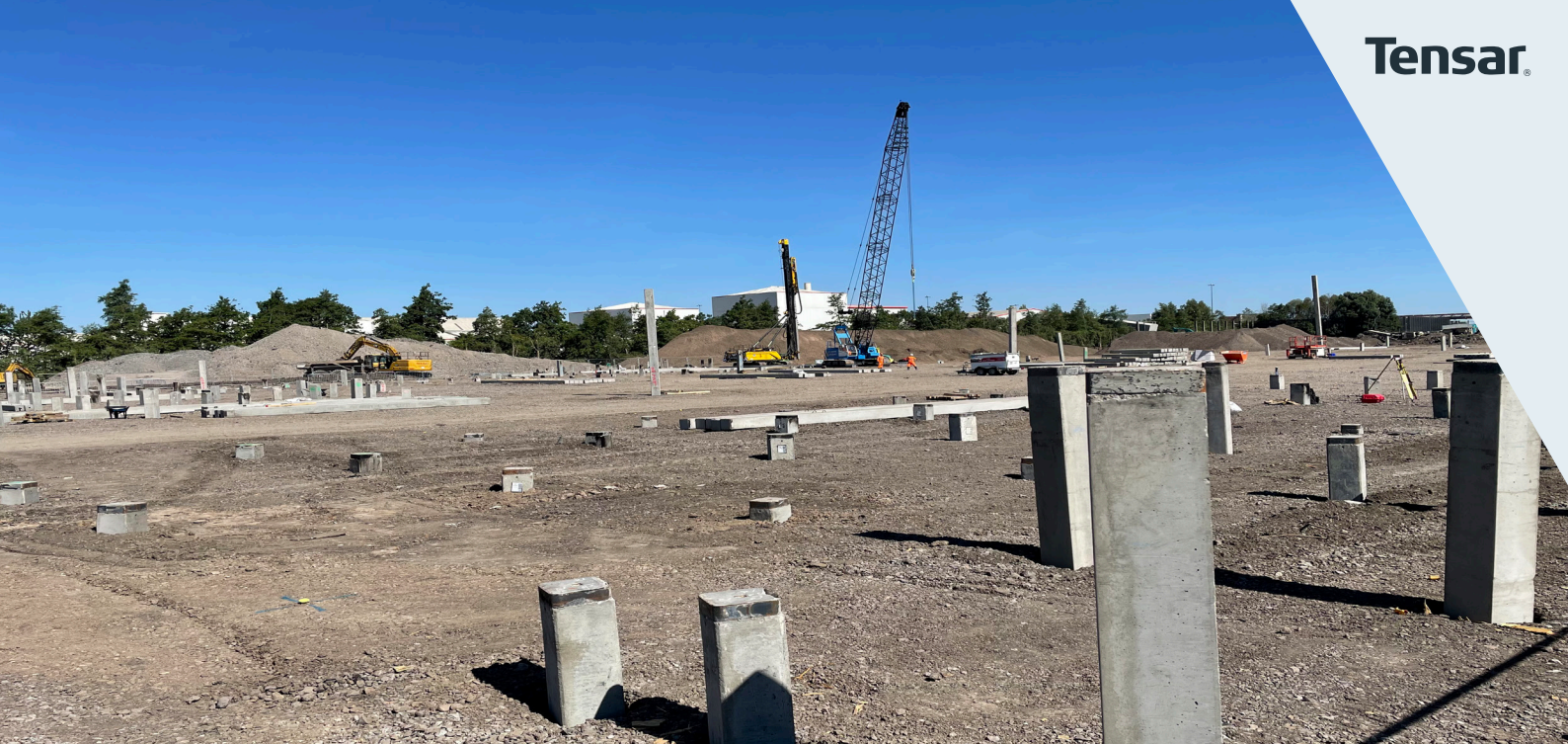
Concrete piles up to 14m in depth, driven through the Tensar mechanically stabilised working platform
