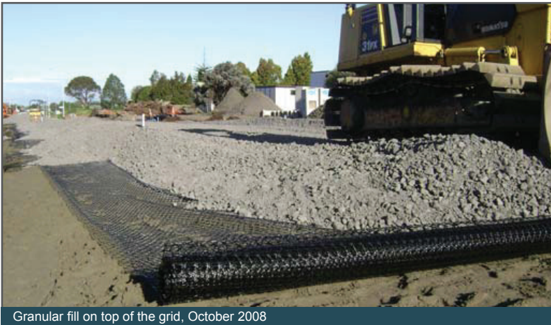
Granular fill on top of the grid, October 2008
