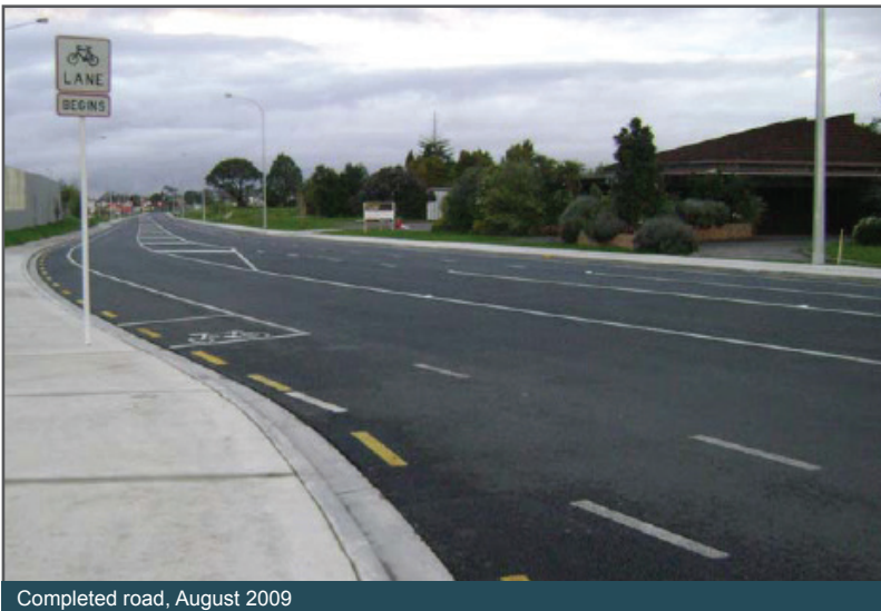
Completed road, August 2009
