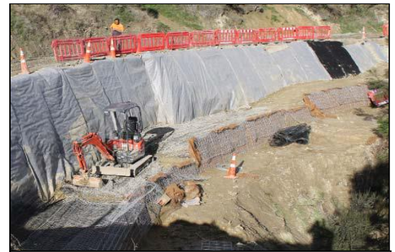
Construction of Green Terramesh wall
