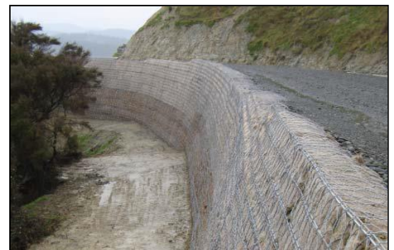
Constructed Green Terramesh wall
