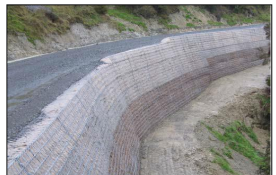
Close up view of completed wall
