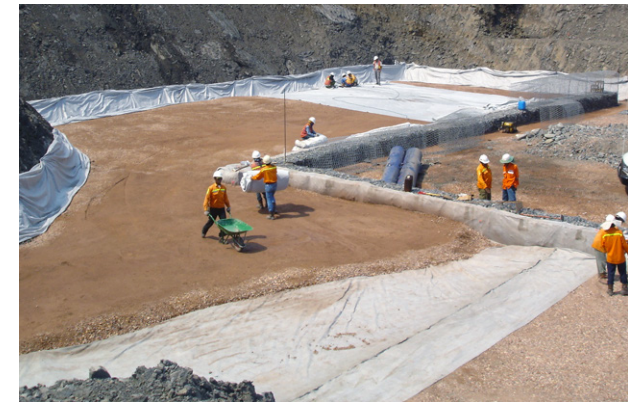
Placing MIRAFI Polyfelt PEC geocomposite across reinforced soil wall
