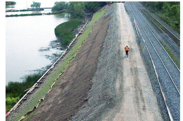
Installation of erosion control mats prior to vegetation
