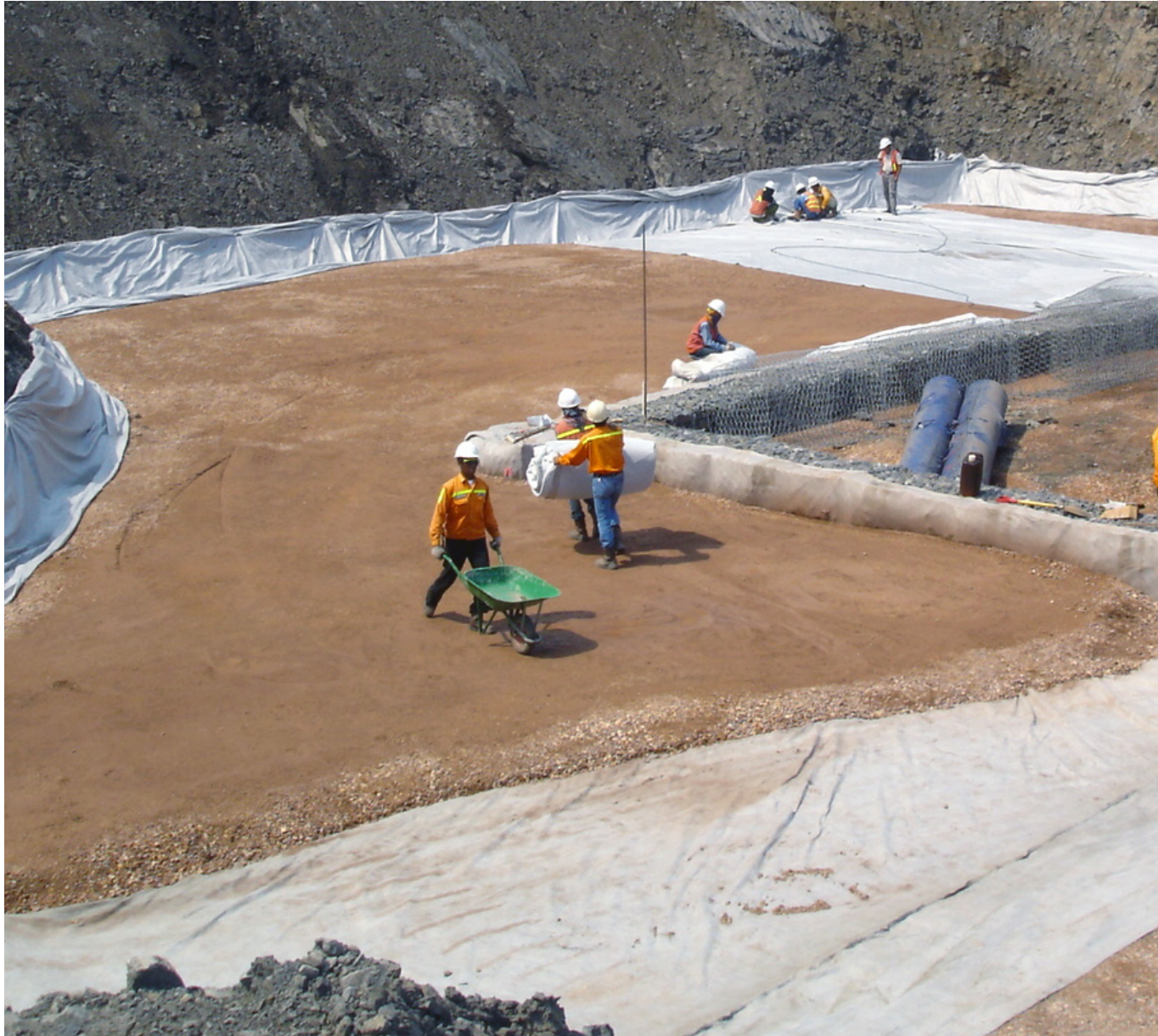
Placing MIRAFI Polyfelt PEC geocomposite across reinforced soil wall
