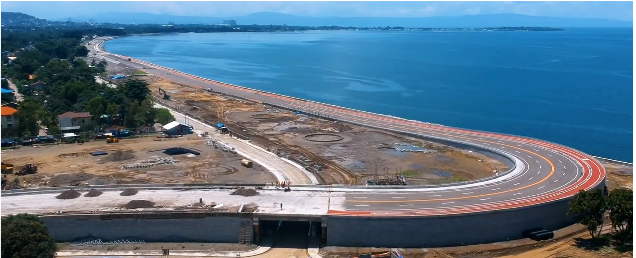
Back to back mechanically stabilized earth wall at bridge abutment
