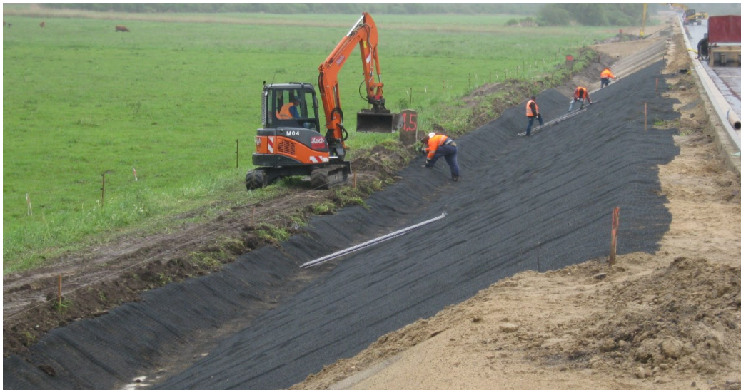
EnkaMat on dry slopes of embankments and earth structures
