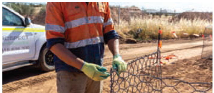
Fig. 6 – Raising panels into position
