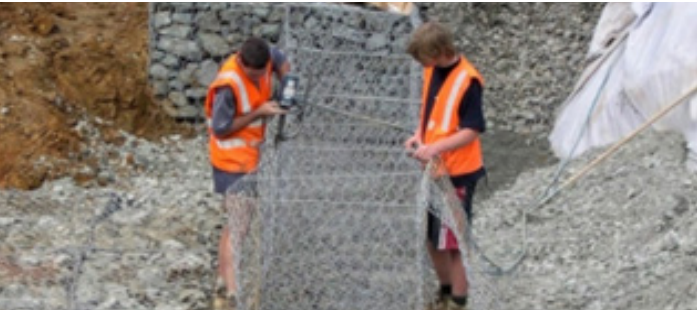
Fig. 7 – Connecting diaphragm
