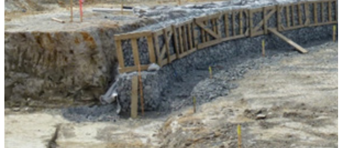
Fig. 4 – Prepared foundation
