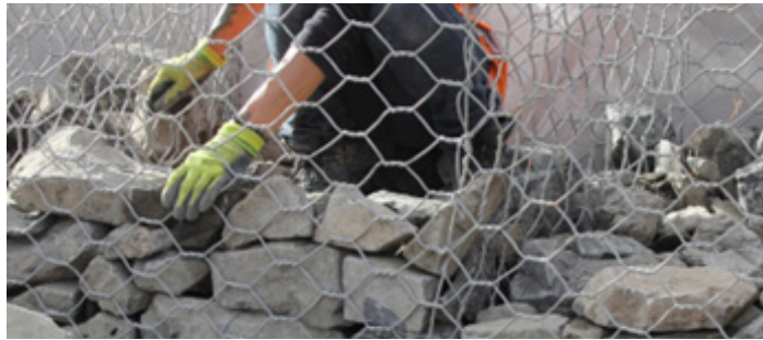
Fig. 13 – Hand stacking stone in front face
