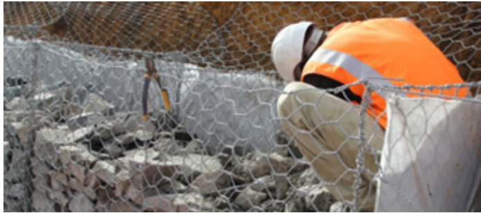
Fig. 11 – Installing bracing wire
