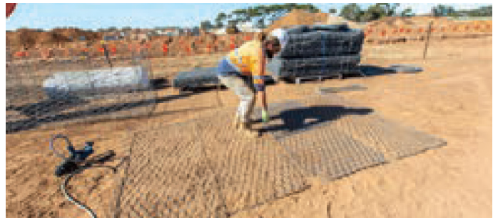
Fig. 5 – Flattening gabion
