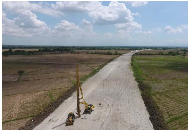
Installation of Alidrain® PVD over soft clay foundation to accelerate consolidation.
