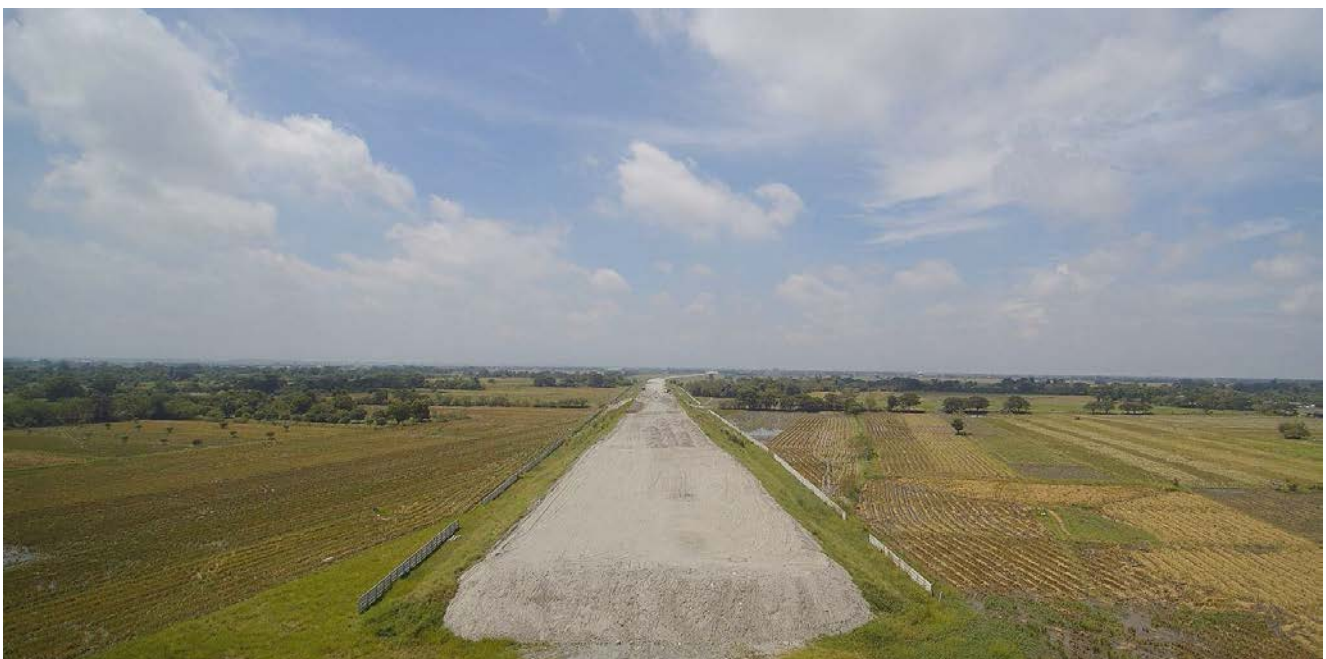
Embankment fill over consolidated soft clay foundation
