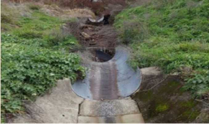
Before the project commenced
