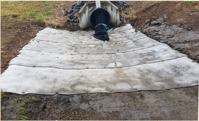
Concrete Canvas weed suppressant and drain outlet finished project
