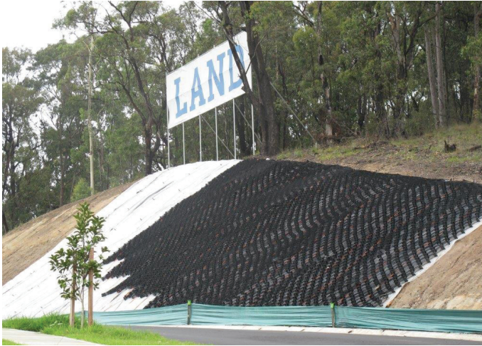
INSTALLATION OF THE GEOWEB SYSTEM ON THE SLOPE
