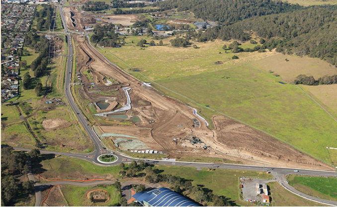
Albion Park Rail Bypass construction photos - June 2019
