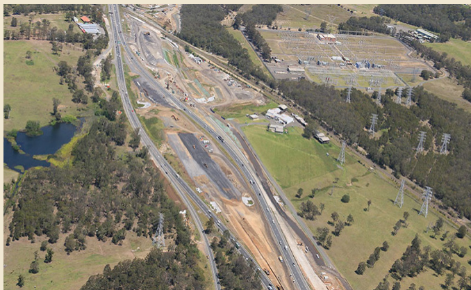
Albion Park Rail Bypass construction photos - October 2019
