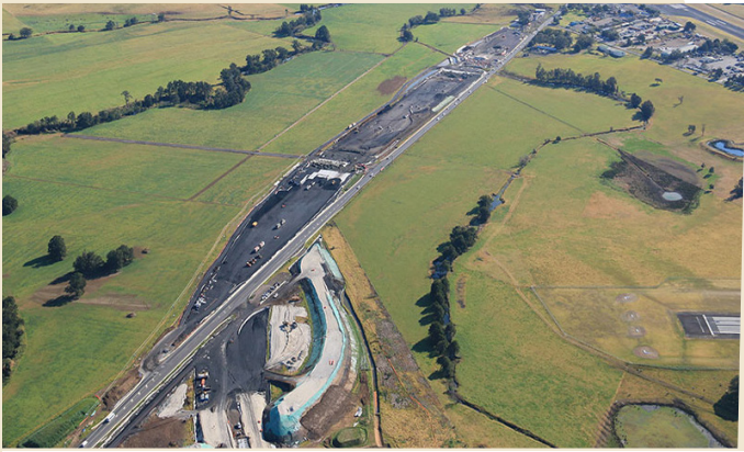
Albion Park Rail Bypass construction photos - August 2019
