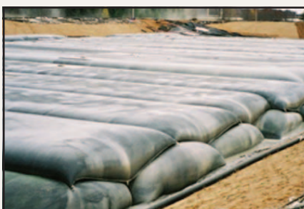
Geotube® containers in activated sludge basin at paper plant.
