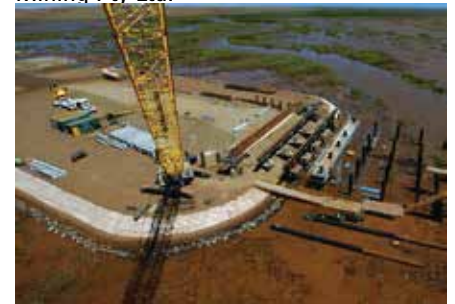
Construction of basal reinforced causeway abutment
