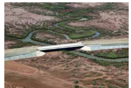
Completed reinforced causeway and bridge structure
