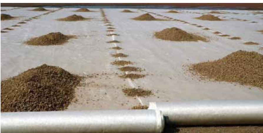
Layout of Mirafi® PET800-50 woven geotextile reinforcement on site
